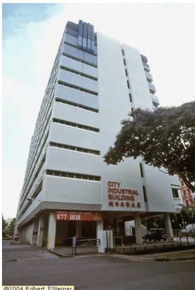
City Industrial Building
