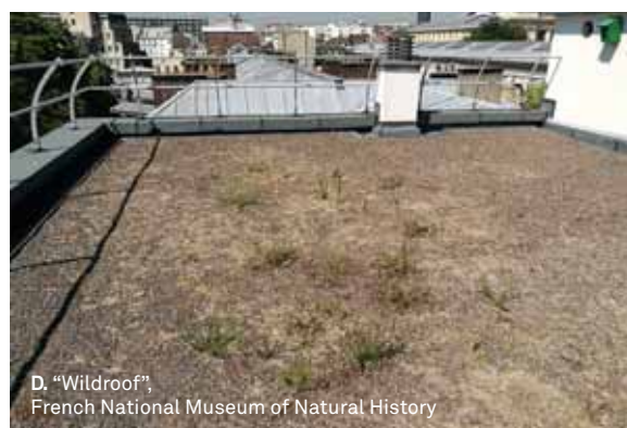
FIGURE 4 Typology of green roofs used in the GROOVES study, based on the definition used by the designers of green roofs. © ARB idF | Institut Paris Region
