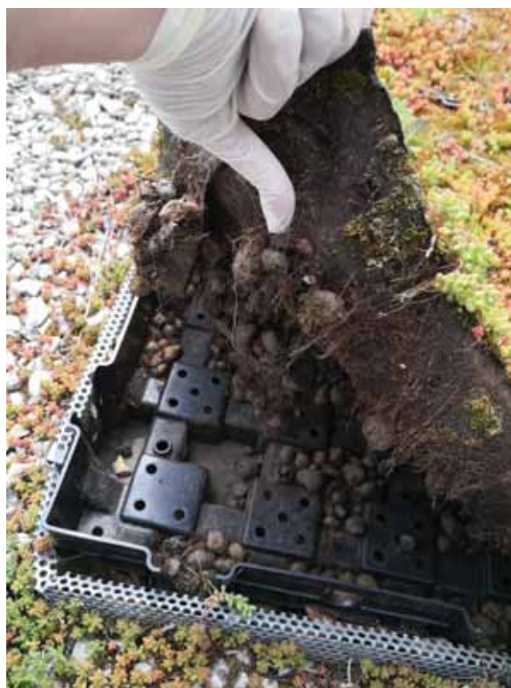
Some planting systems decay and can leave traces behind. Avoiding the use of plastics is more essential than ever in the design of green roofs. © Marc Barra | ARB idF
