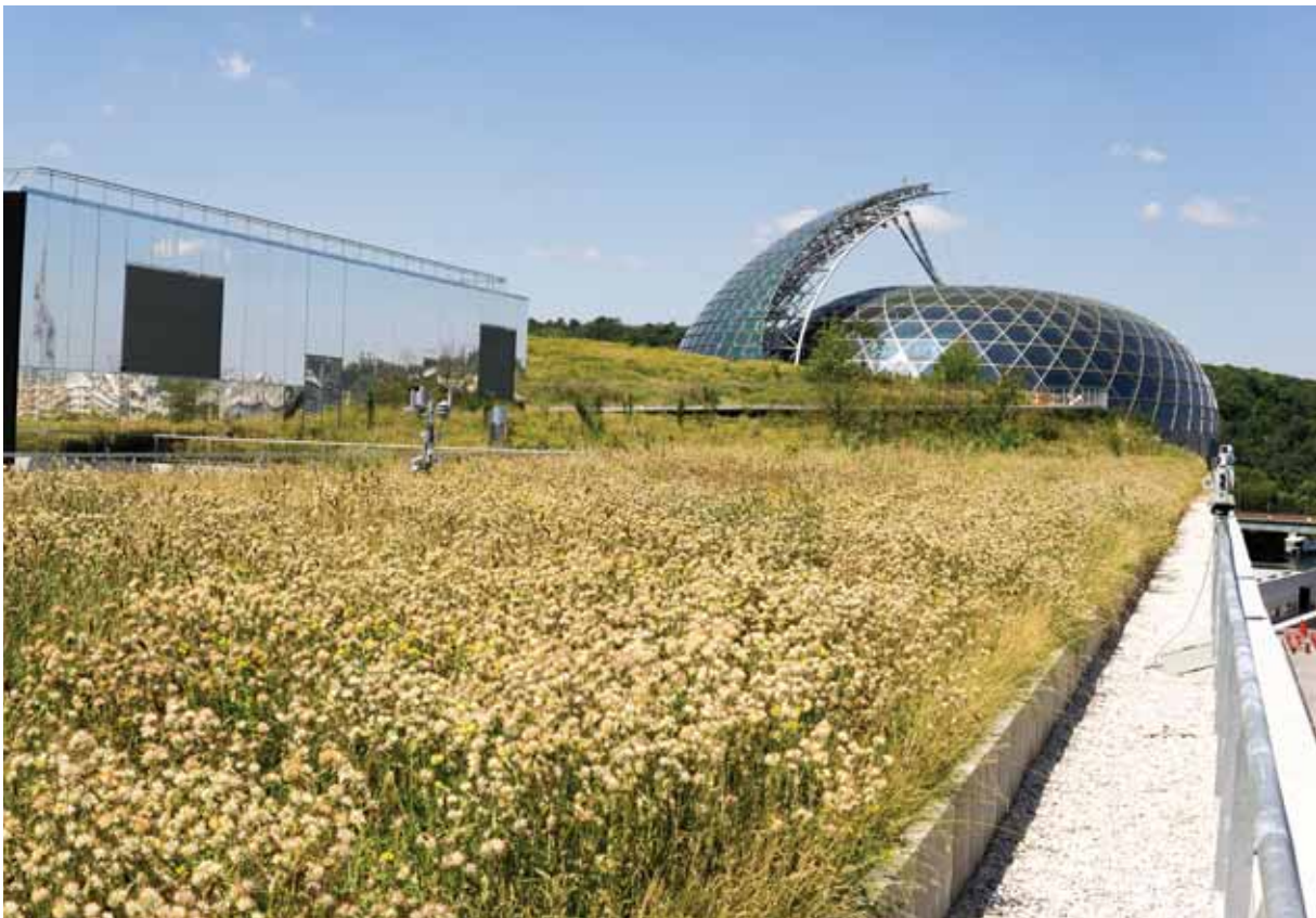
The roof of La Seine Musicale in Boulogne-Billancourt has a water retention capacity of about 184 L/sq.m. © Audrey Muratet | ARB idF
