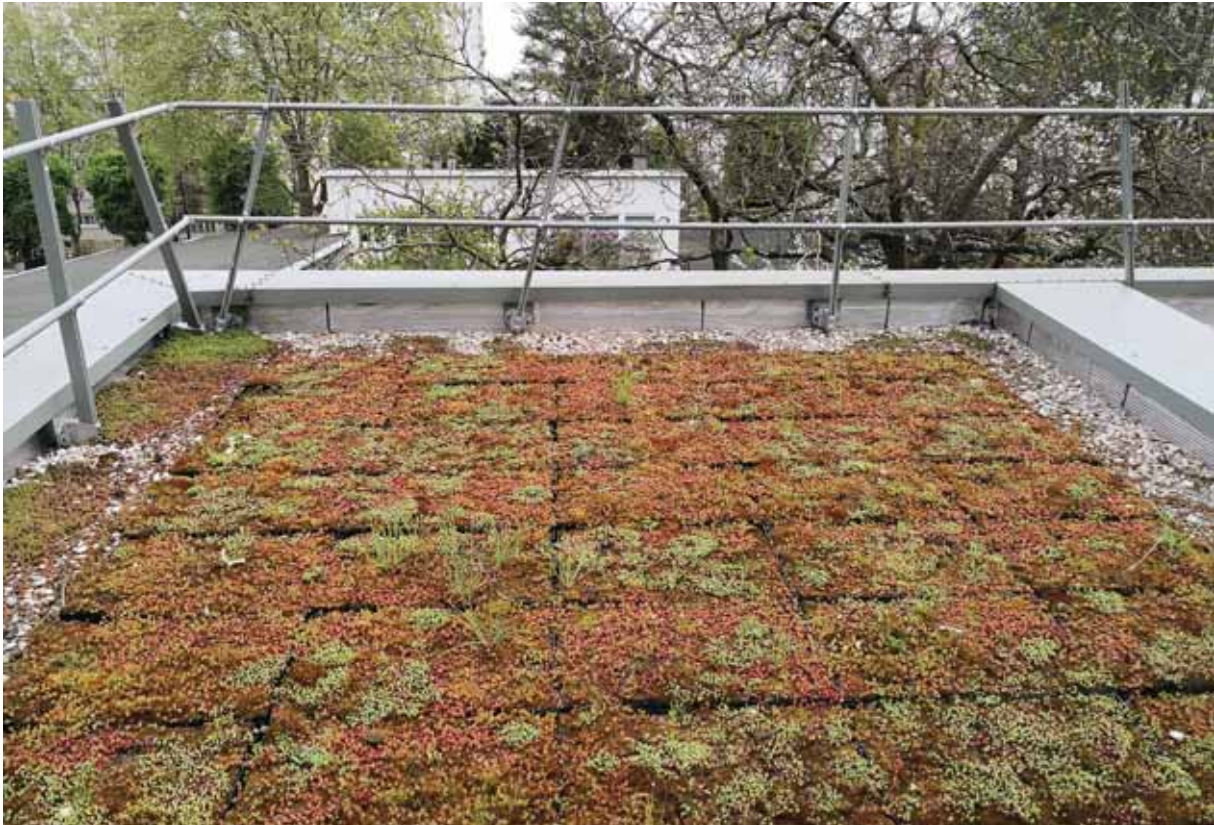
Green roofs are often sold in the form of factory-packed plants. A Life Cycle Assessment (LCA) may be necessary to evaluate their overall impact © Marc Barra | ARB ïdF
